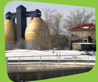
Back River Wastewater Treatment Plant in Baltimore, MD
