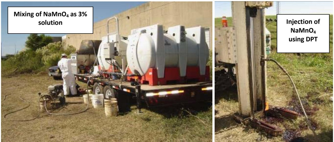
**Figure 4:** Direct injection of soluble  $\text{NaMnO}_4$ .
