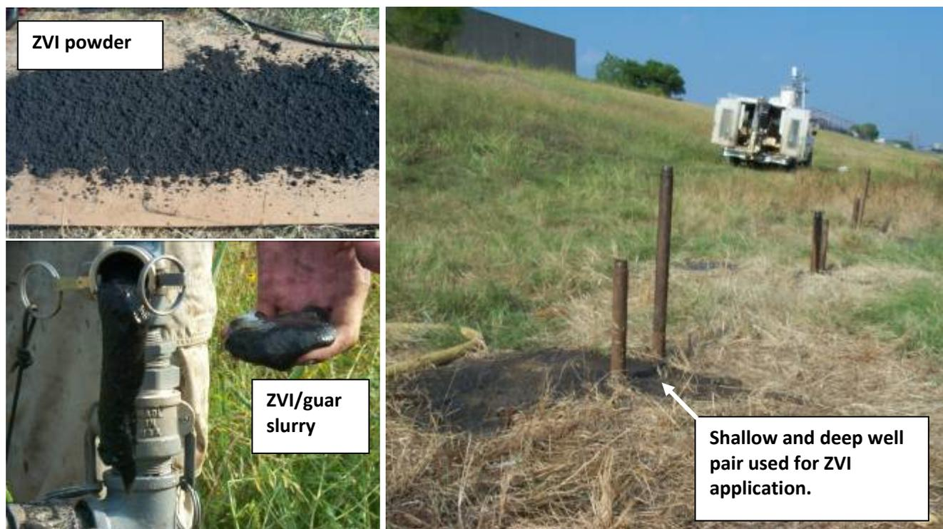
**Figure 5:** ZVI injected as a guar slurry using hydraulic fracturing applied via injection wells.
