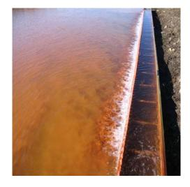
Due to the high volume of water coming out of the mine and to maximize its potential; the design also had to incorporate a segregated gate so it wouldn't allow any water to pass by and could be cleaned out periodically. Additionally, a notched weir was incorporated to control the volume of fluid which passed through with a weir flow rate @ full 2" head pressure @ 48.6 cubic feet per second.
