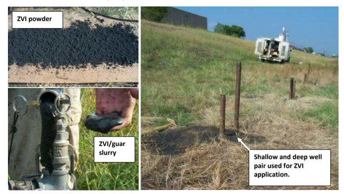
**Figure 5:** ZVI injected as a guar slurry using hydraulic fracturing applied via injection wells.
