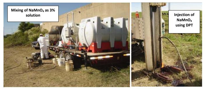
**Figure 4:** Direct injection of soluble NaMnO<sub>4</sub>.
