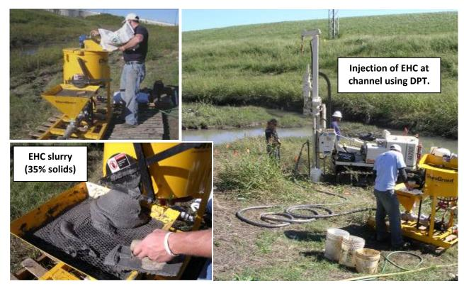
**Figure 6:** Injection of EHC at channel using DPT. Preparation of EHC slurry containing 35% solids using Chem Grout's CG-550 mixing system.
