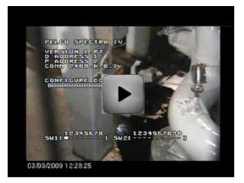
**Figure 2:** In this oil spill, the operator was not notified until the floor in the pumping station was inches deep in fuel oil, and the leak detector finally went off. Observing the video absolved the operator, because it became obvious that the leak detector was in the wrong place.
